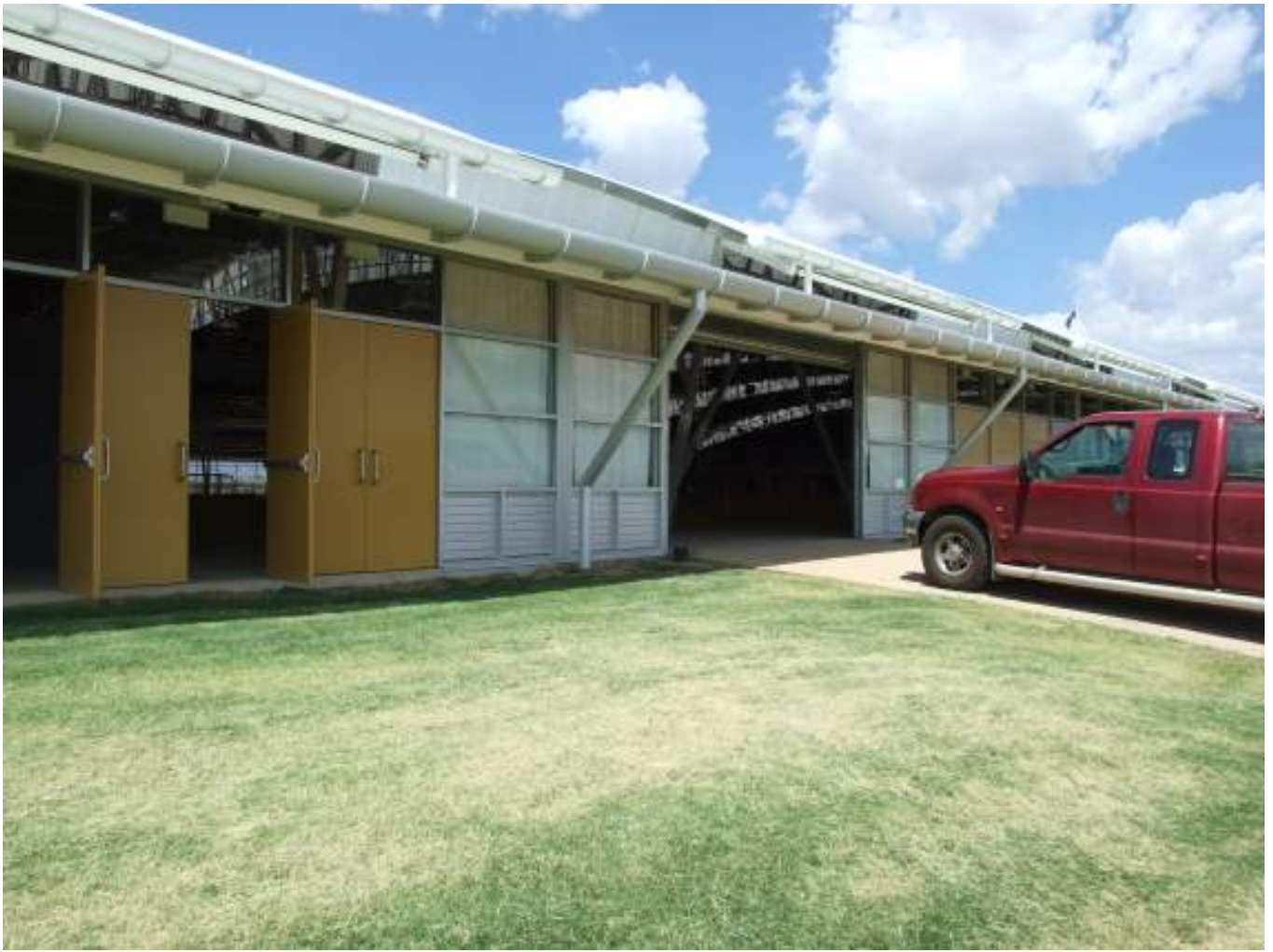
AELEC – Roller Door Entry – Traders are able to drive light vehicles onto the concourse level to load/unload
